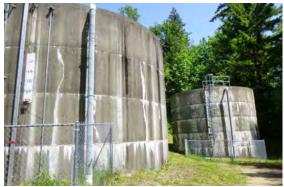
The water system is supplied by two concrete storage tanks. Our understanding is these tanks are original and even though there is evidence of water leeching the tanks appear to be well maintained and reportedly have regular interior and exterior inspections.
